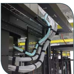
Side access for cable zones
